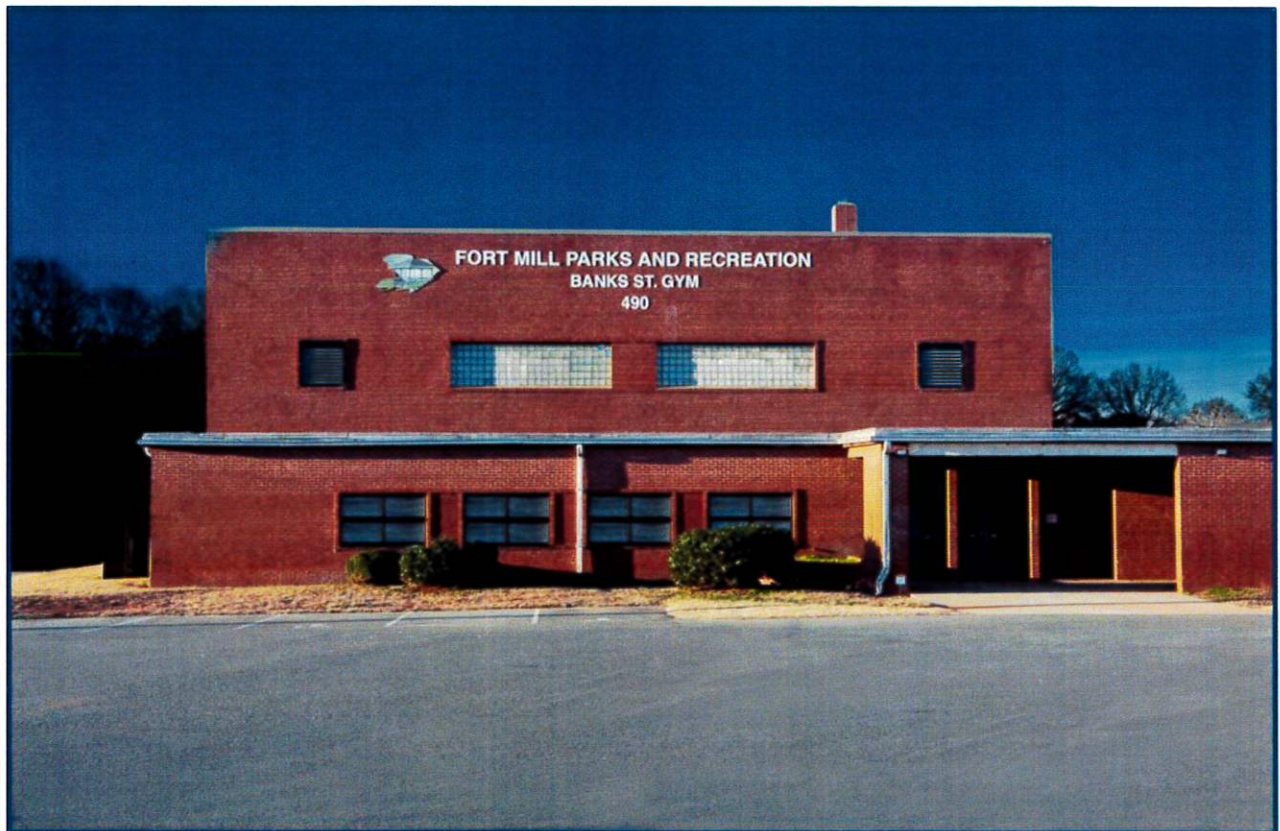
Existing Facade - Fort Mill Community Center
